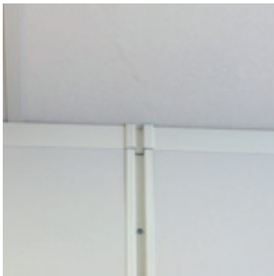
Detalj mot himling.
